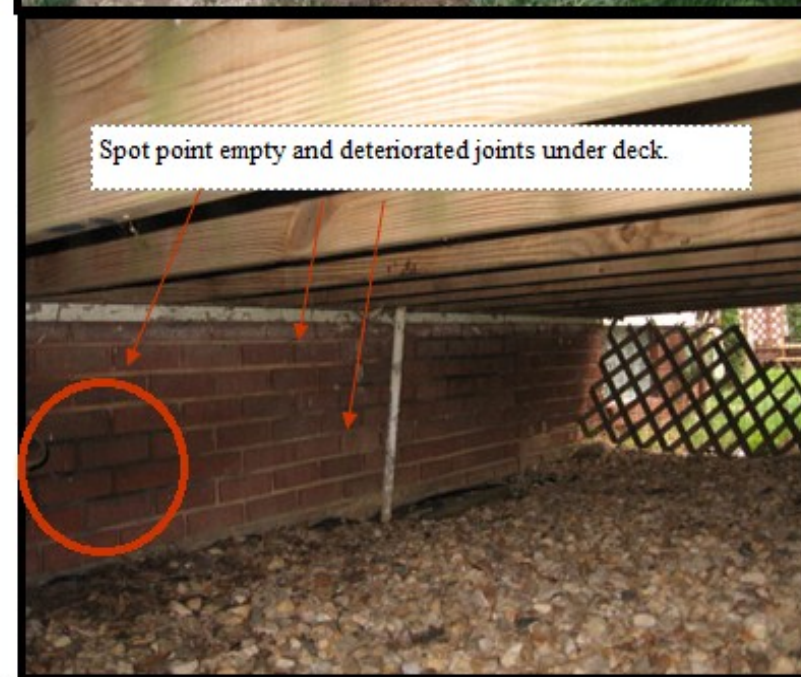
West side of house to the north of chimney. Example of joints that would be spot pointed.
