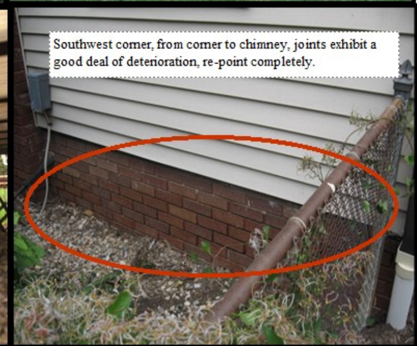
Southwest corner, from corner to chimney, joints exhibit a good deal of deterioration, re-point completely.
