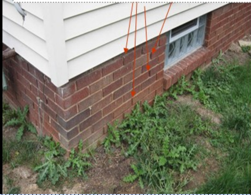
Northwest corner of home example of empty joints that would be
