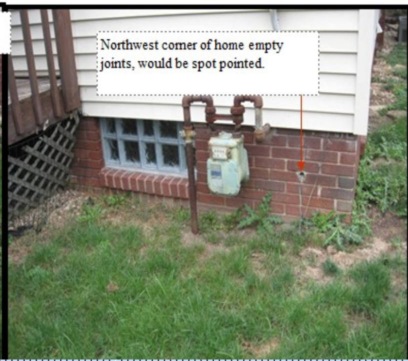
Northwest corner of home example of empty joints that would be
