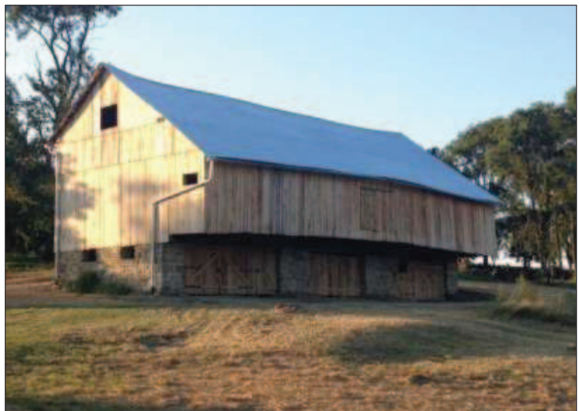
View of southeast oblique of barn after rehabilitation work was complete.
