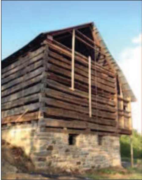
View of southwest corner during work..
