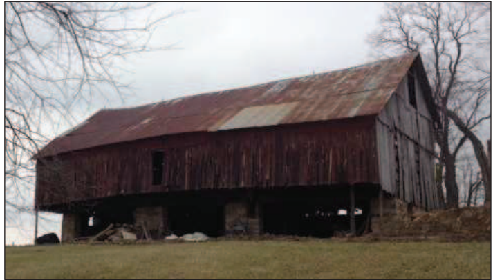
Northwest oblique of Curtis' barn before rehabilitation, Somerset, OH. All photographs by author.
